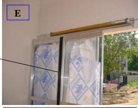
Hang right side track ( track without Operator ) as shown in Figure F (This track will be flush with track shown in Figure E)
